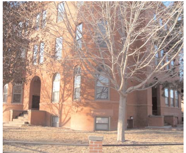
Campion House, the new home for Institute offices, is located on the corner of 19th and California streets.
